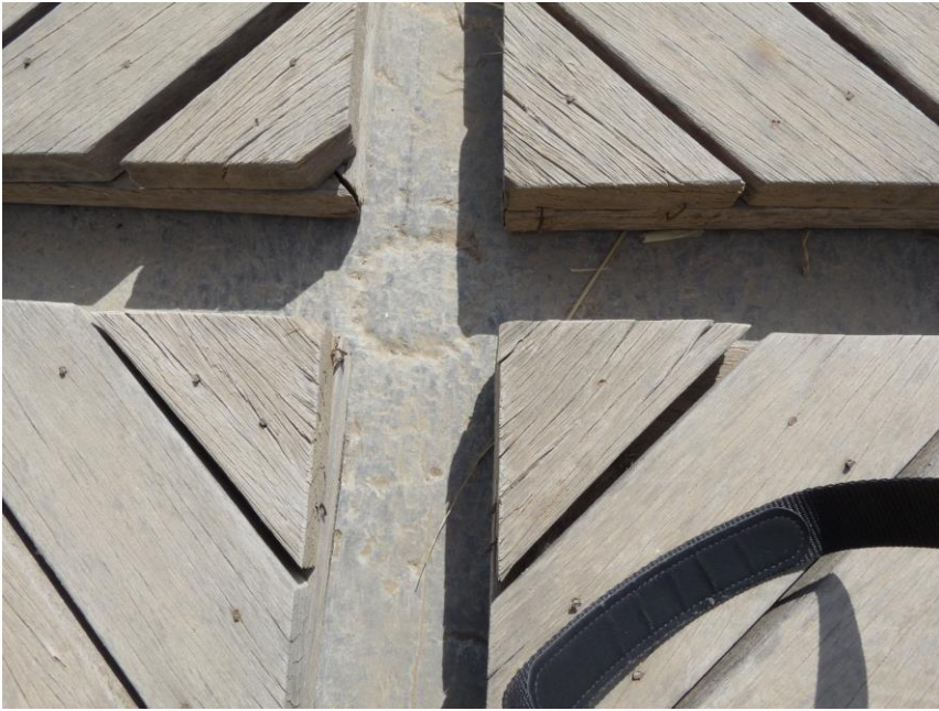
Pedastal of the pillar at Persipolis (covered by wodden plank to avoid damage)
