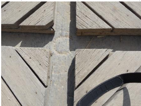
Pedestal of the pillar at Persepolis (covered by wooden plank to avoid damage)
